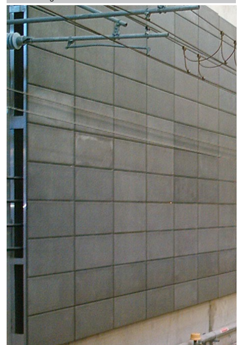
During Installation. Aluminium framework is still visible.
