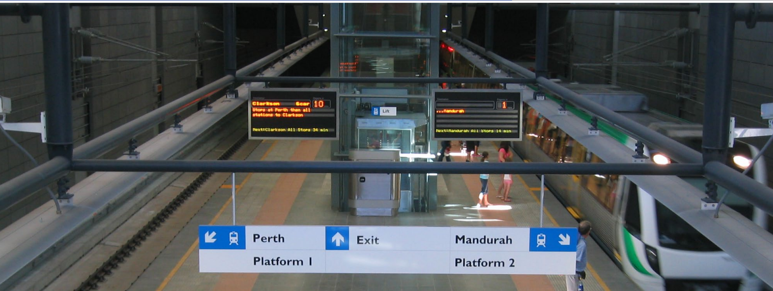
Quietstone wall panels are clearly visible down either side of the rail tracks.
